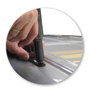
While holding the permanent mount block firmly on roof, rivet the blocks to the roof.
