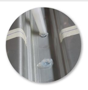
Apply neutral cure silicon sealant in and around drilled holes.
